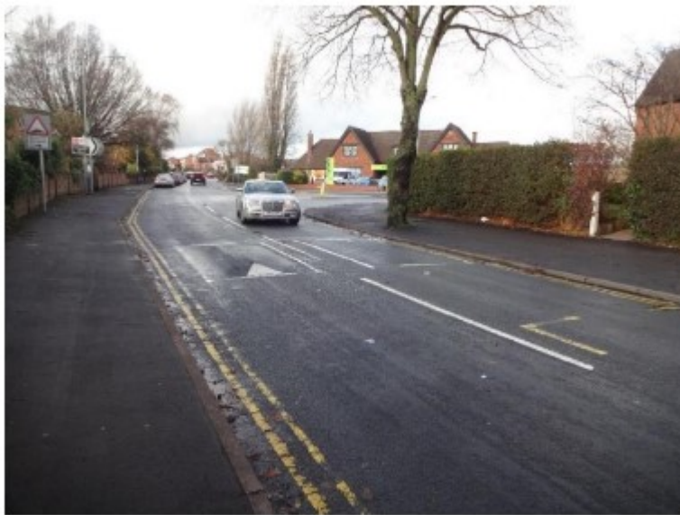
Speed cushions, Cape Road, Warwick
